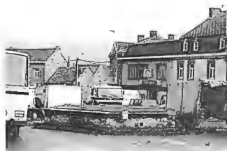
5. Comblain-au-Pont, place Leblanc
